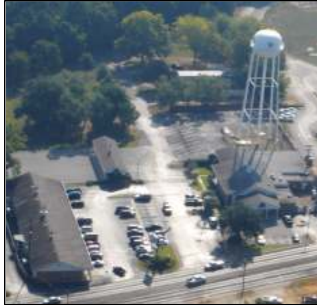
Image 9.18: The Austin Bank complex and other Town Center commercial development along Horton Street
