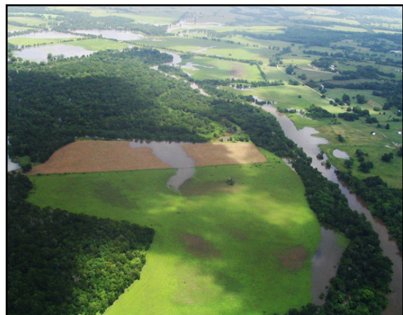
Navasota River Flooding
