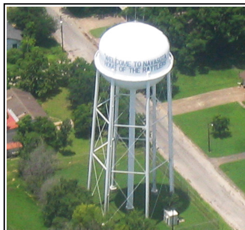
0.4 MG Elevated Water Tower
