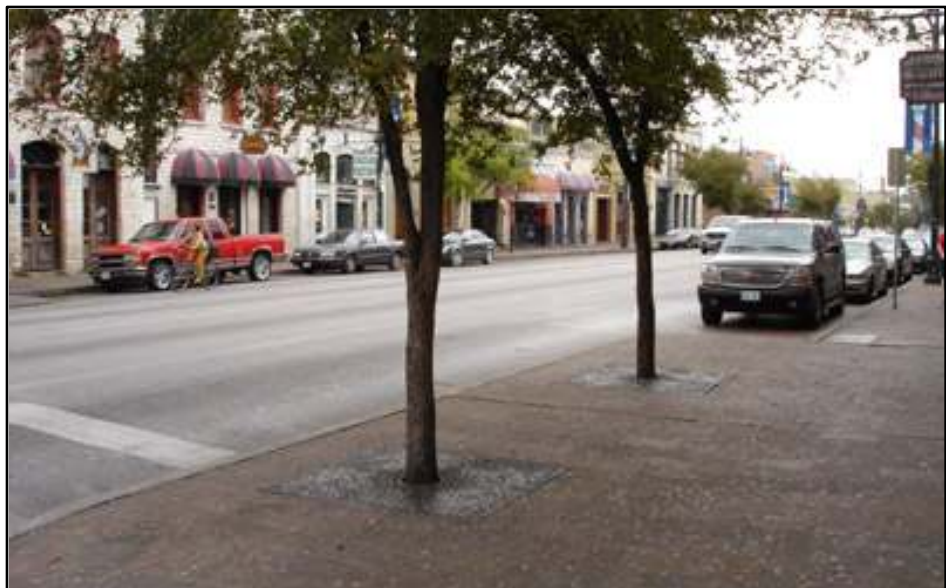
Image 4.4: Bulb out in Downtown Austin, TX with young street trees and brick paving
