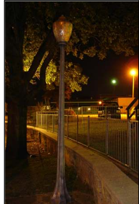
Image 4.11: Mixed bulb types and burned out fixtures are found throughout Downtown
