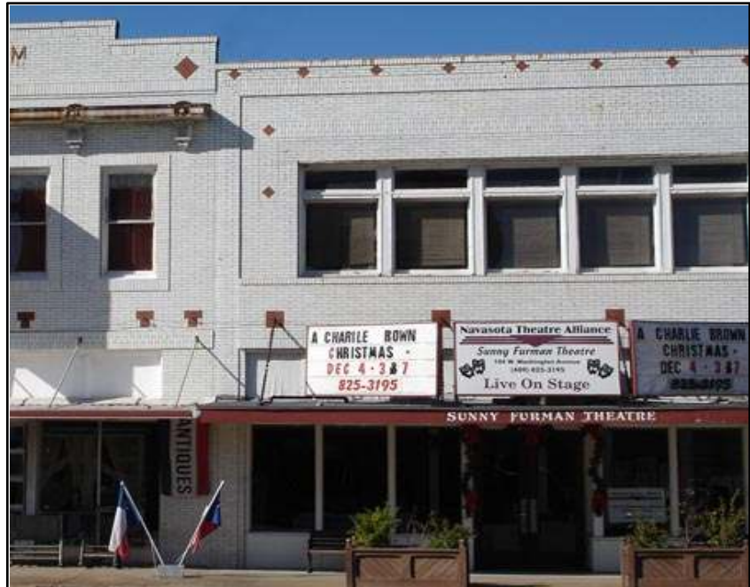
Image 3.4: The Sunny Furman Theatre generates parking demand on an irregular basis but can cause major impacts during performances on surrounding parking groups throughout Zone 4
